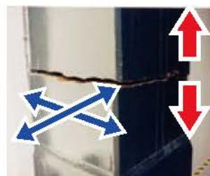
柱の破断 (1995 Kobe Earthquake)
