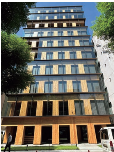
Fig. 1 Port Plus-11 Story Pure Wood Building in Yokohama
