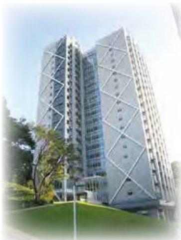
地震・風観測を行っている超高層免震建物 (すずかけ台キャンパス) High-rise Isolated Building where Earthquake and Wind Observation are Carried out in Suzukakedai Campus
